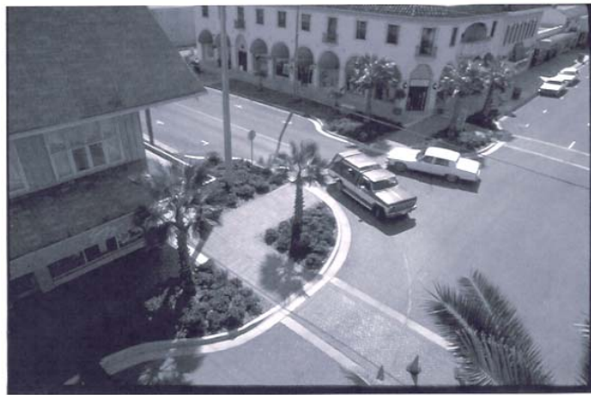
A bulb-out at an intersection reduces the time it takes pedestrians to cross the street, preserves the curb lane for parking, and serves as a traffic-calming device. (Courtesy of Dan Burden, Walkable Communities, Inc.)
