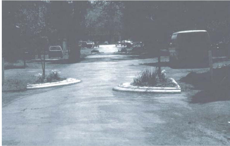
A choker on a two-way roadway narrows the street and serves as a traffic calming device. (Photo courtesy of Dan Burden, Walkable Communities, Inc.)
