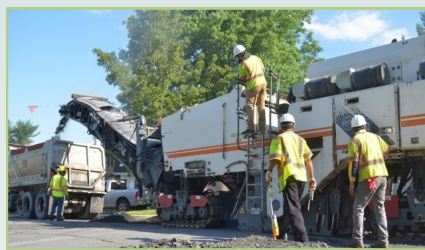
Typical milling operation
