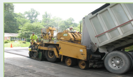
Typical hot mix asphalt paving operation
